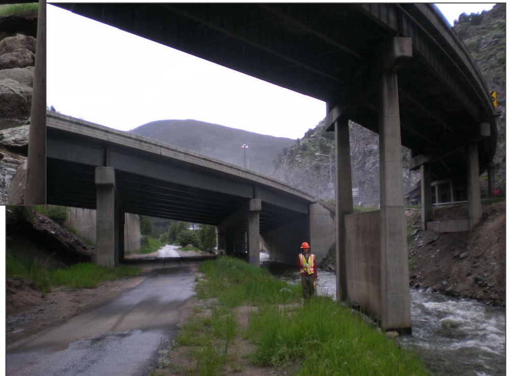
Clear Creek/ US 6 Interchange
